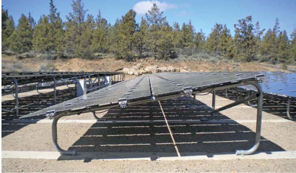
In areas with no vegetative growth or snow shed, racks can attach to concrete at ground level.
